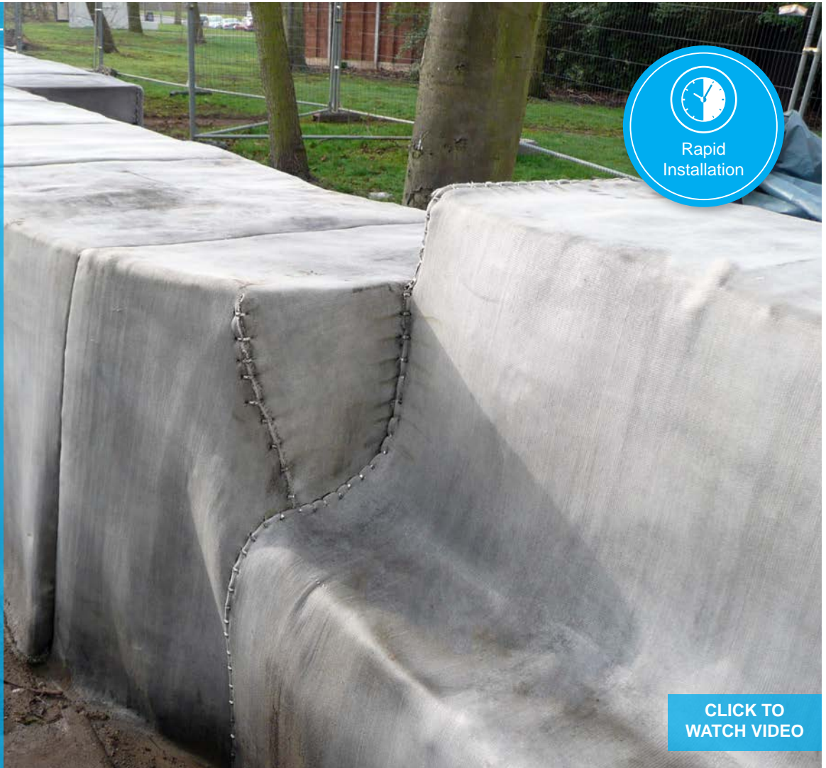
Completed CC lined gabion section
