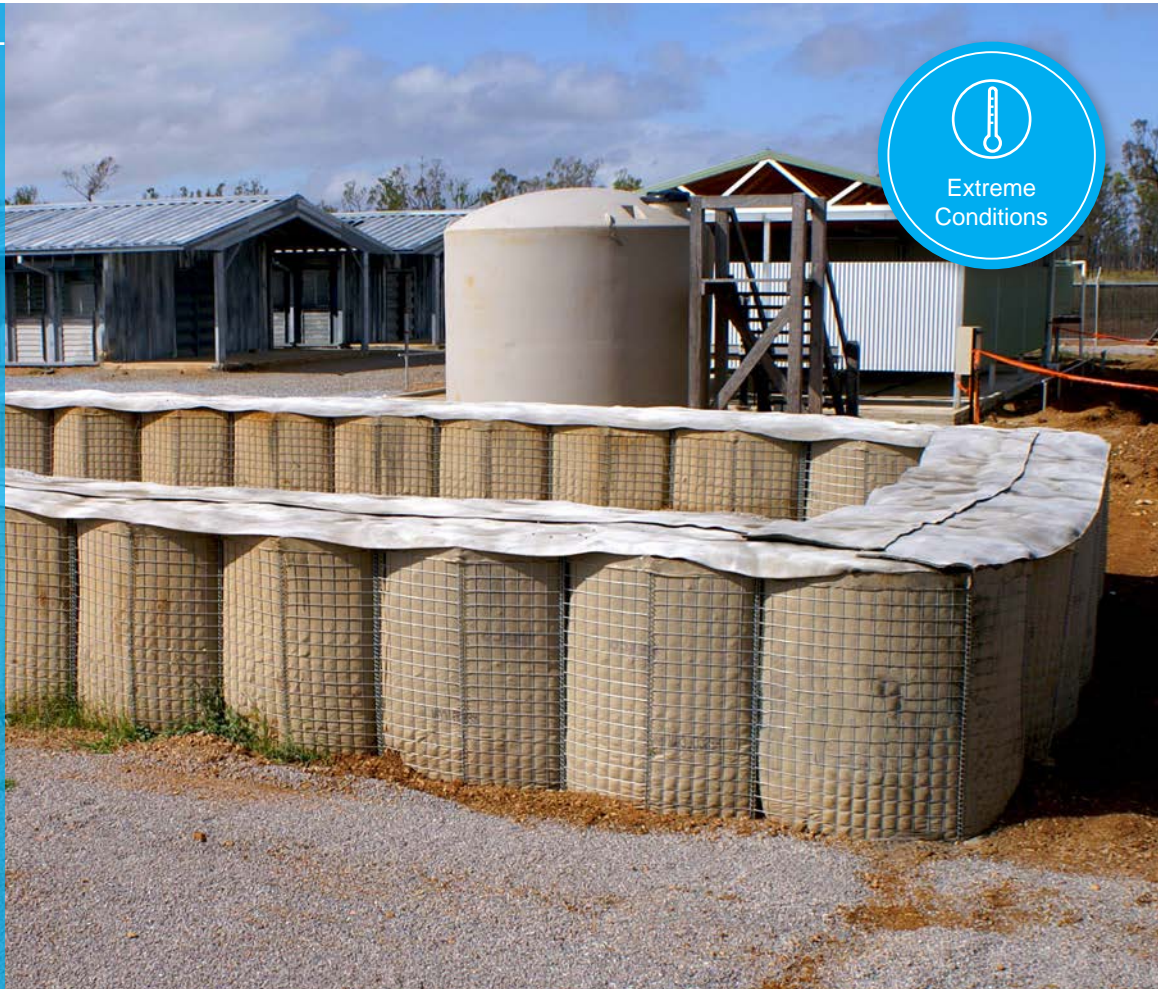
Completed gabion capping
