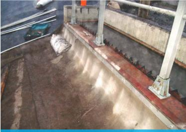
CC fixed to inlet structure using CT1, hammer screws and GRP batten
