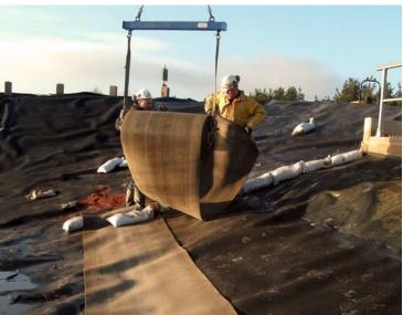
CC bulk rolls deployed from excavator using spreader beam
